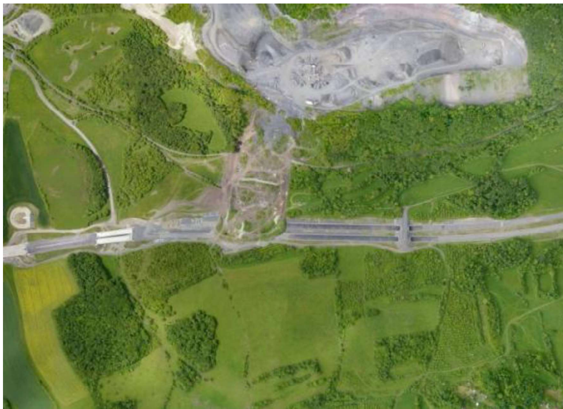
Figure 4. Extensive landslide in the D8 motorway area (2013) [4]
